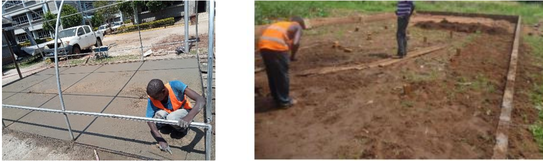
Figure 21: Foundation concrete slab laying
