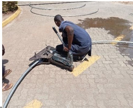
Figure 15: Bending of the hoops/arches using hydraulic pipe bender
