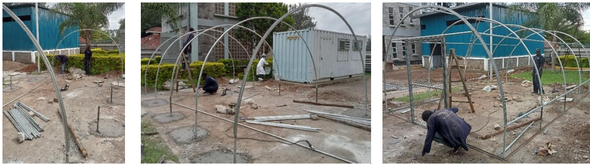
Figure 22: Construction of super structure
