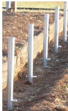
Figure 20: Installation of other foundation pipes
