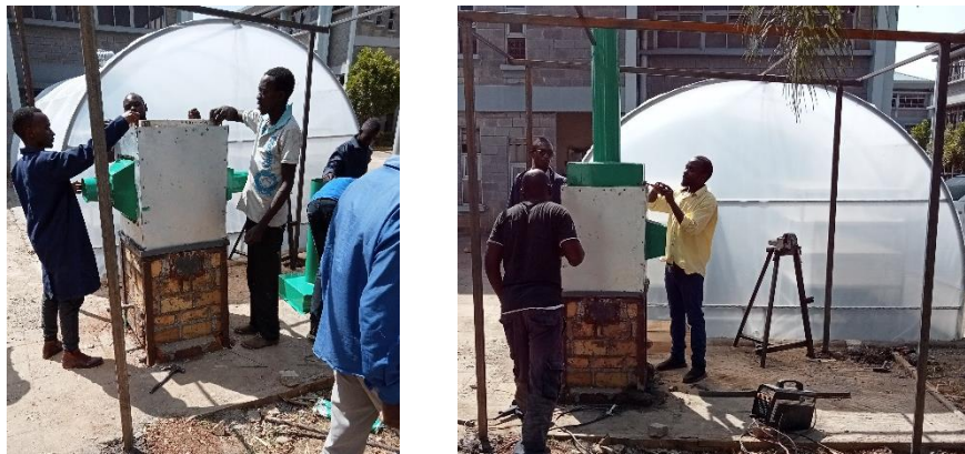
Figure 28: Assembling of Biomass heat exchanger system
