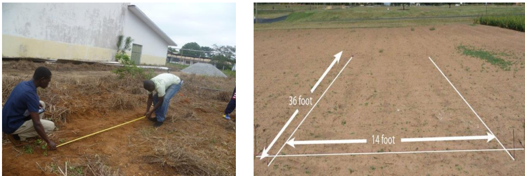
Figure 16: Measurement and marking out construction area
