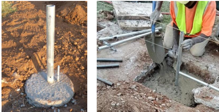
Figure 19: Corner pipes covered with concrete
