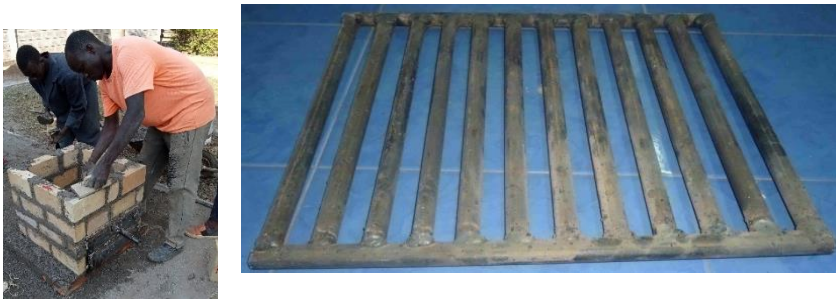
Figure 27: (a) Construction of biomass furnace (b) Grate design
