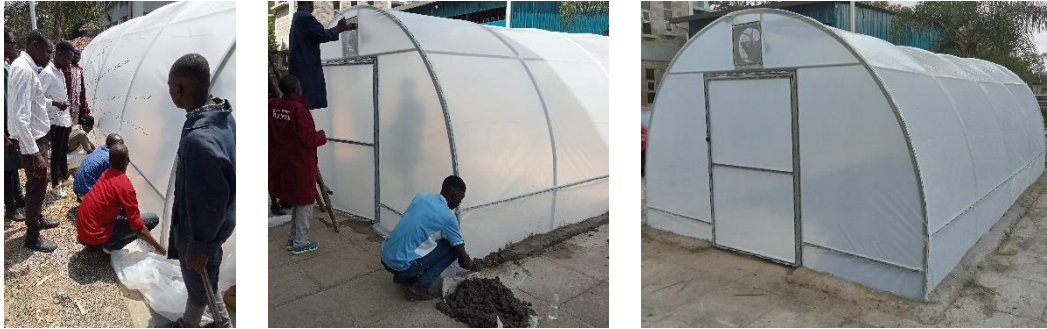
Figure 23: Cladding or covering of drying chamber
